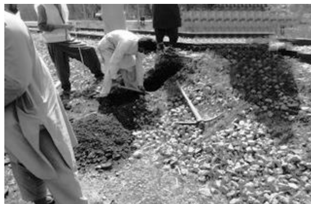
Figure 3: Working on-the site to install Load Cell
